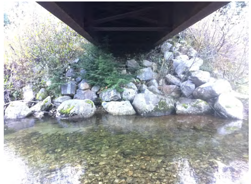
Left Bank Abutment when facing downstream
