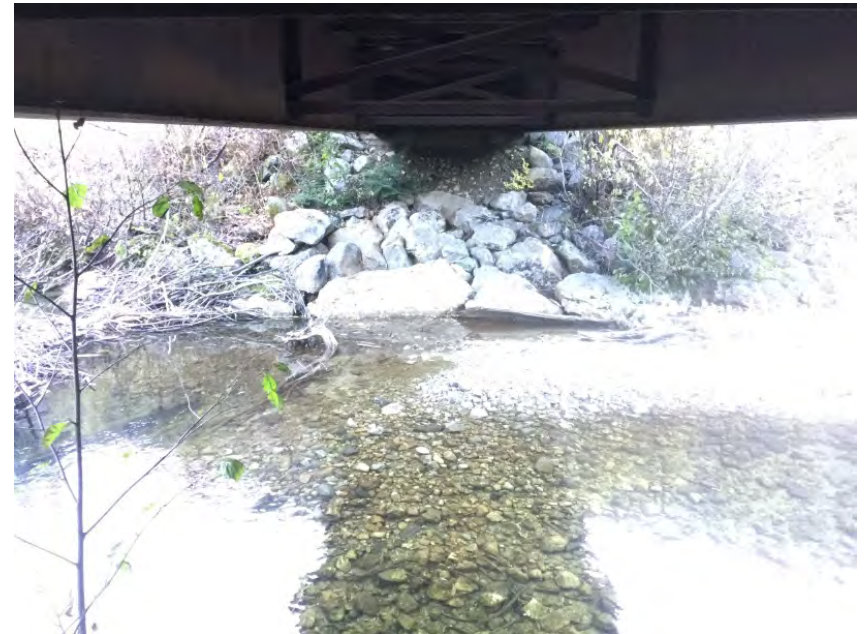
Right Bank Abutment when facing downstream
